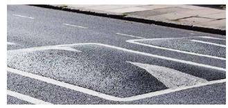
Figure 13: Example of a speed cushion.
