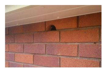
Figure 31: Example of a swift brick under an eave.
